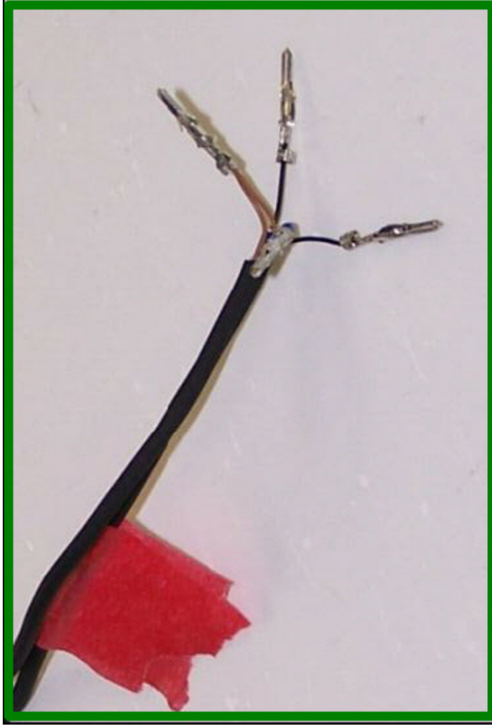
Installed crimp Pins
