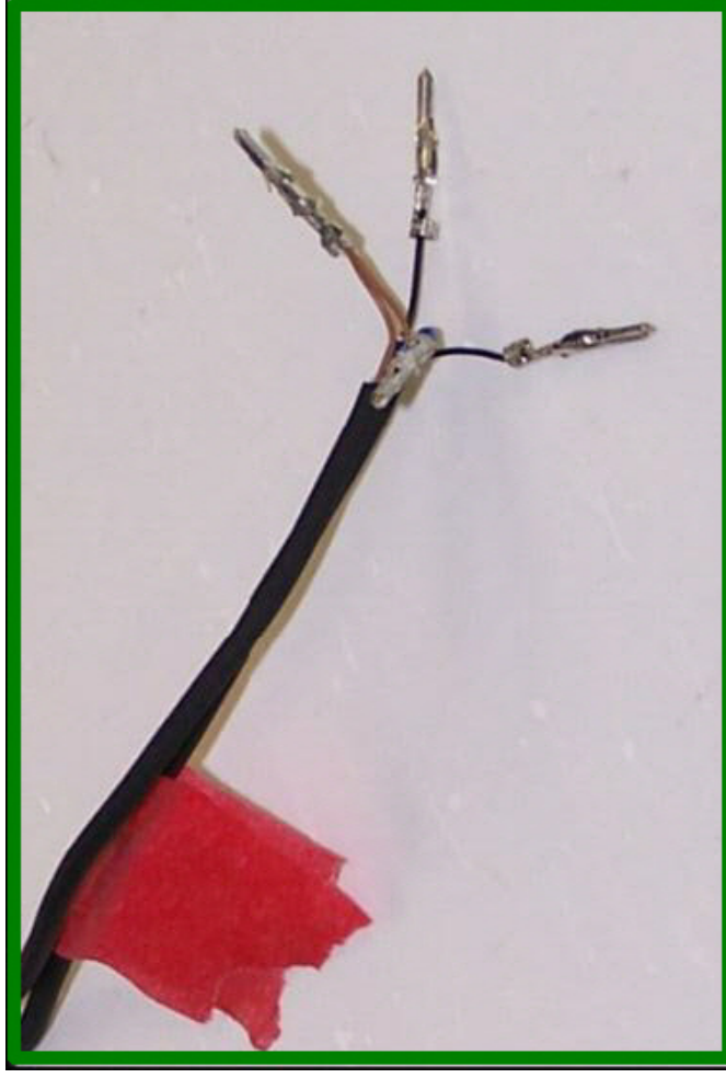
Installed crimp Pins
